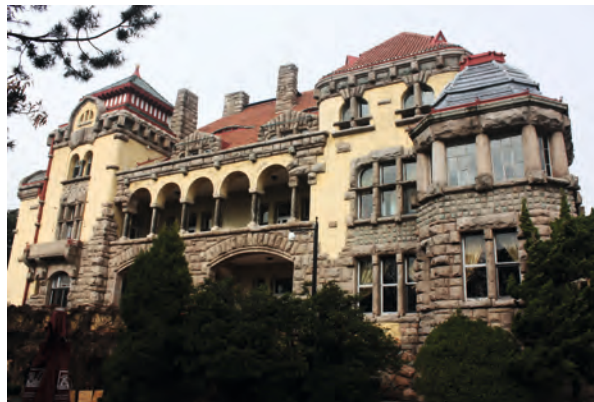
Fig. 3 The former Gouverneurs-Wohnhaus (1905–07) in its present condition (Falser 2018).
